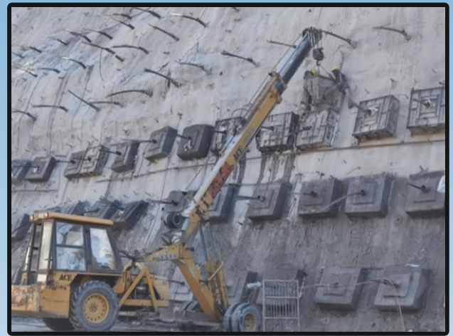
Pre-Stressed Cable Anchor for Slope Stabilization
