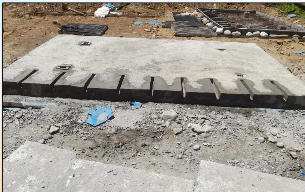
Casting of Precast Pavement Panels in Arunachal Pradesh
