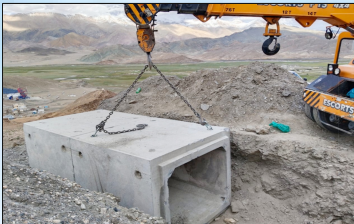
Construction of Pre-cast culvert in Ladakh
