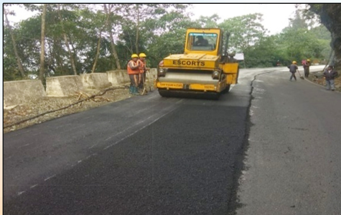
Resurfacing on Phuentsholing-Thimphu Road in Bhutan
