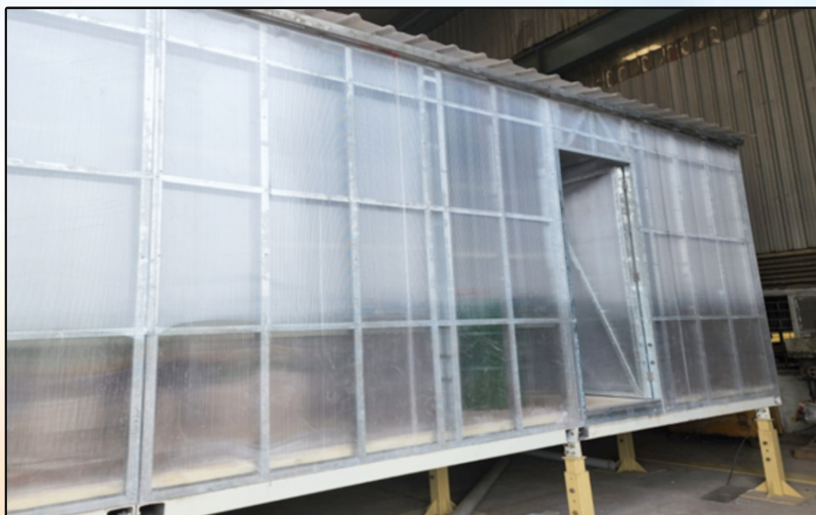
South Facing End for Thermal Gain
