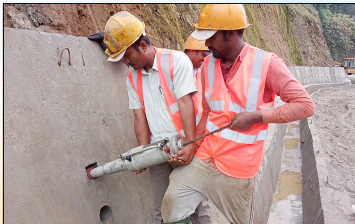
Anchoring Pre-cast Breast Wall on Along-Yingkiong Road in Arunachal Pradesh
