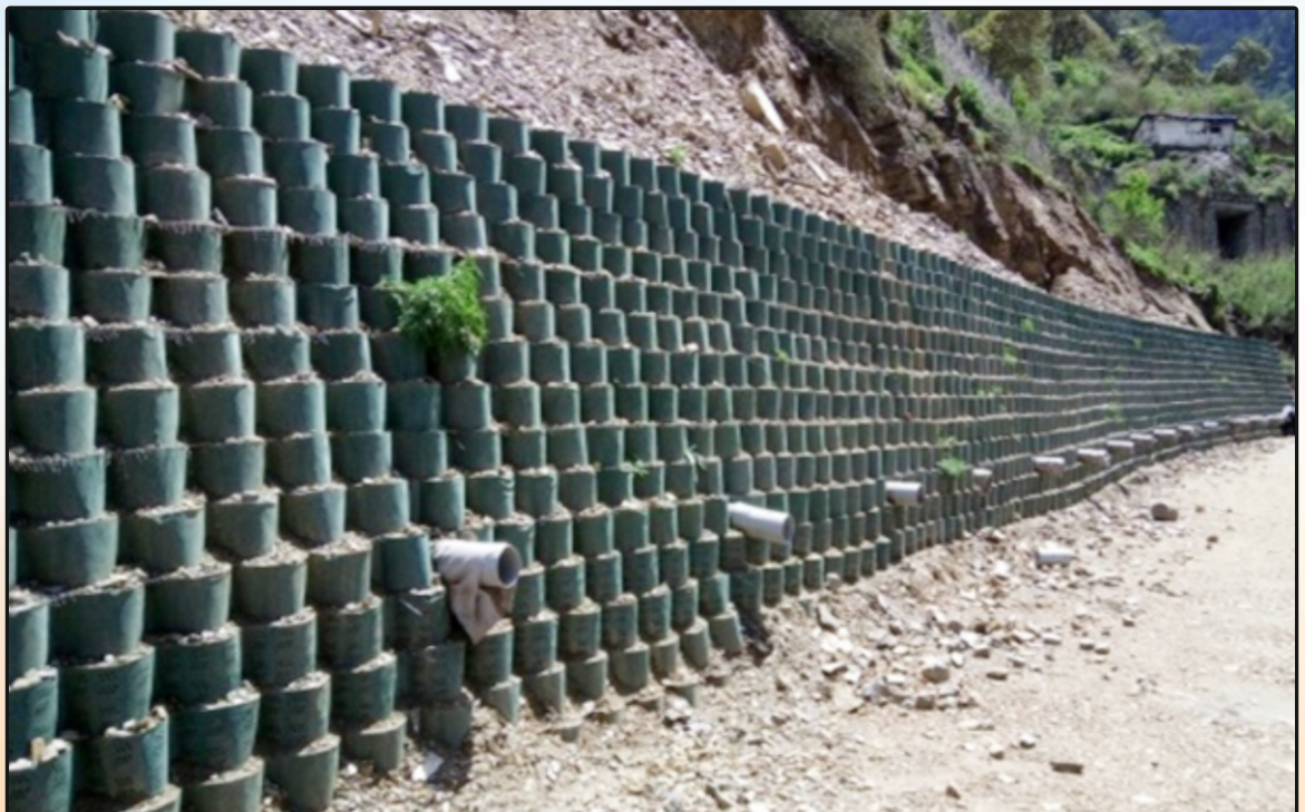
Geo Web on Damchu Haa Link road in Bhutan
