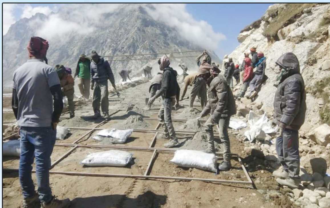
Preparing for Laying CTB Layer on Ghastoli-Rattakona Road in Uttarakhand
