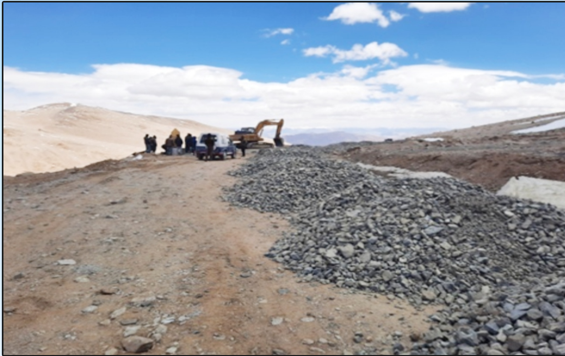
Laying NFSSB Layer on Chisumle-Demchok Road in Ladakh
