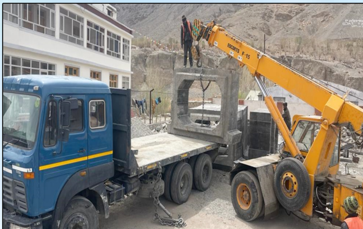
Unloading of Precast Box Culvert Segments in Ladakh
