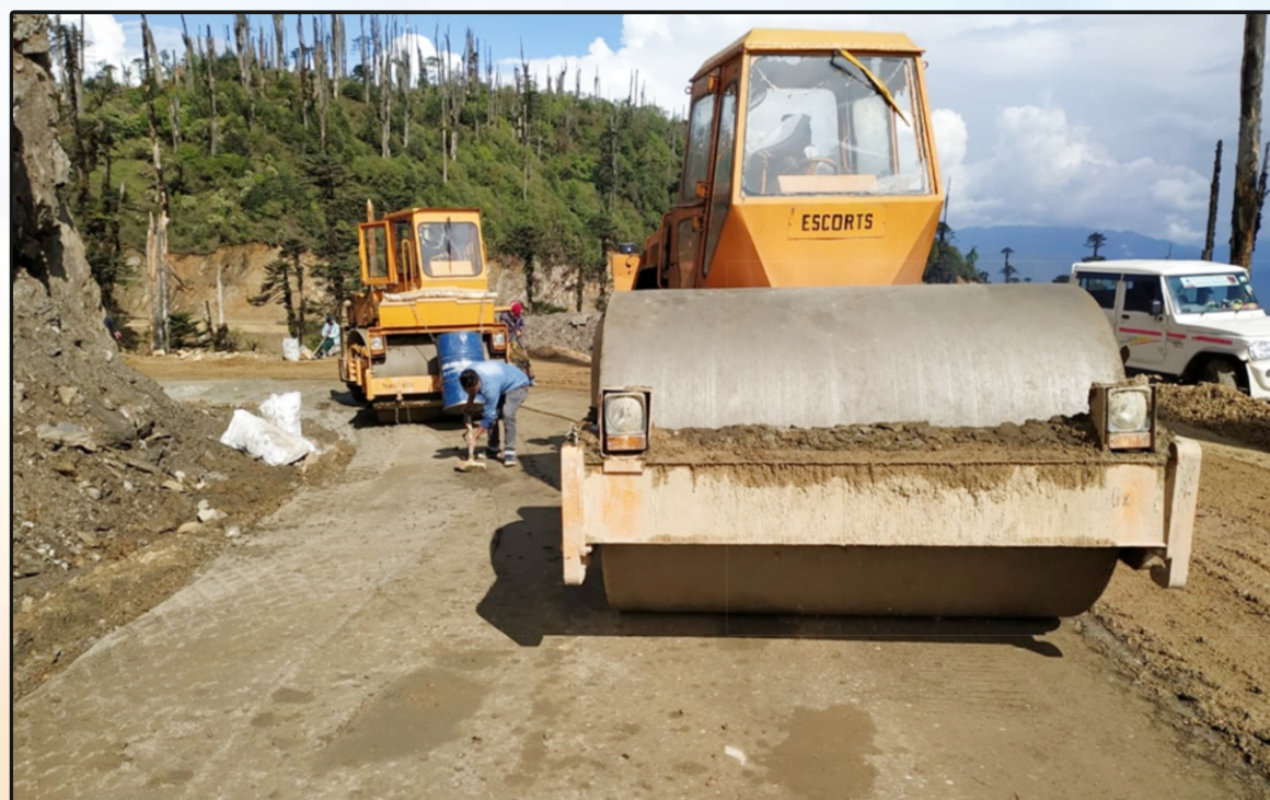
Compacting CTB Layer on Mandala-Debrabu-Naga GG Road in Arunachal Pradesh
