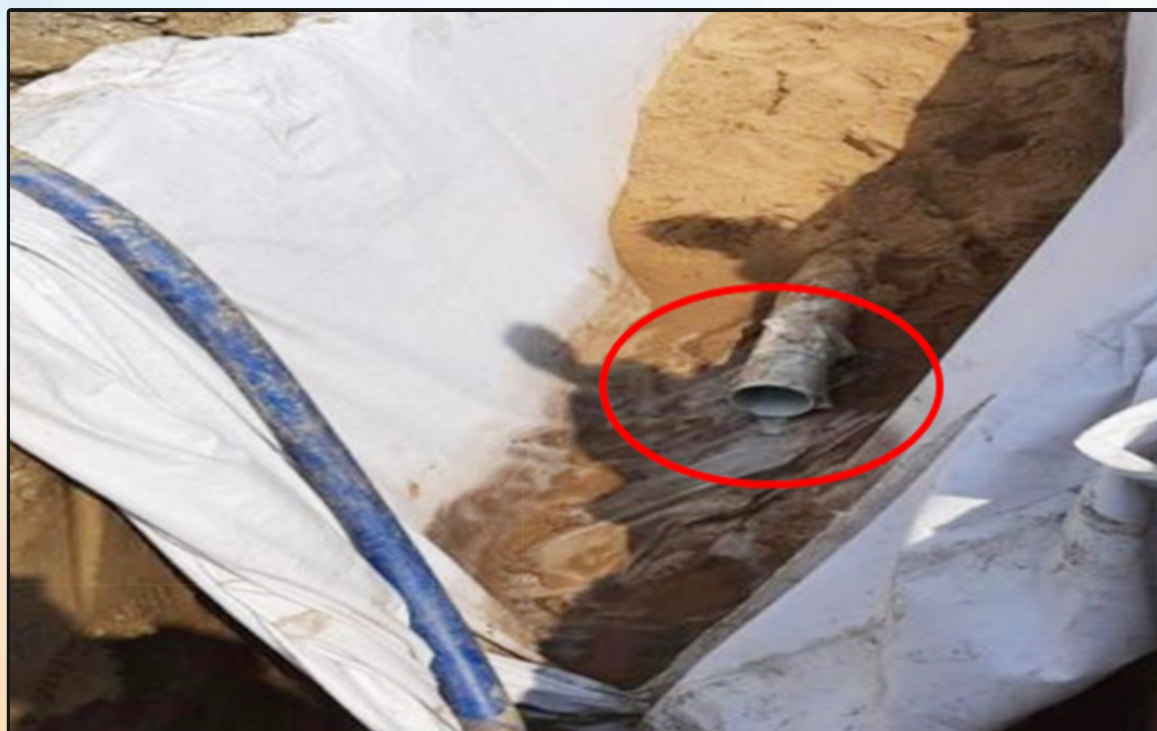
Testing of Sub-Surface Drainage System at Barrackpore Runway in Progress
