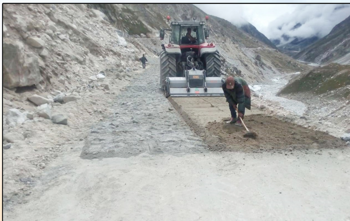
Spreading CT Soil on Ghastoli-Rattakona Road in Uttarakhand
