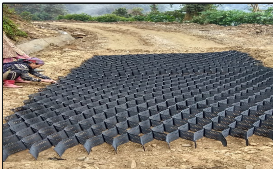
Use of Geocells on Hapoli-Sarli-Huri Road in Arunachal Pradesh
