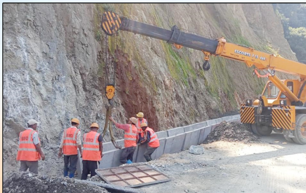
Fixing of Pre-cast Drain on Along-Yingkiong Road in Arunachal Pradesh
