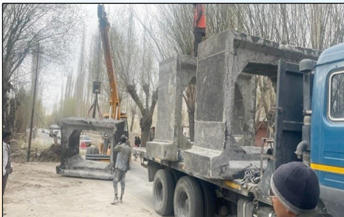
Loading of Precast Box Culvert Segments in Ladakh
