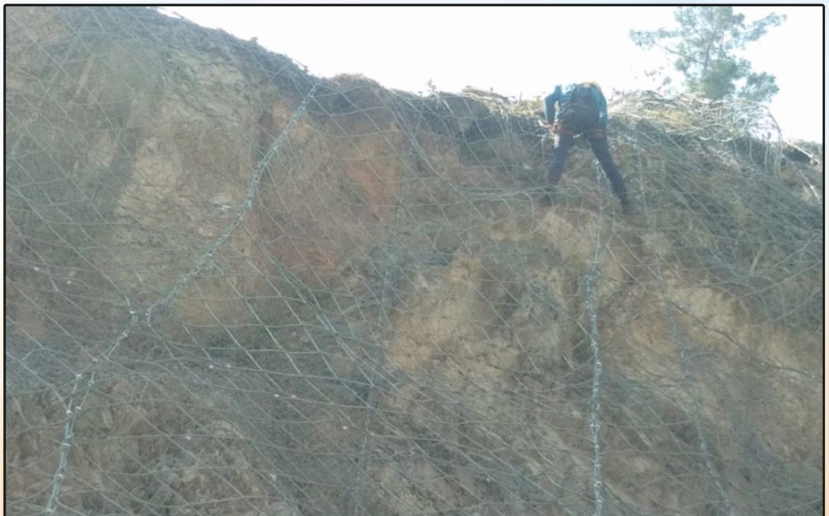
Rock & Bolt Method at Km 144.8 on Orang-Kalaktang-Shergaon-Rupa-Tenga Road in Arunachal Pradesh
