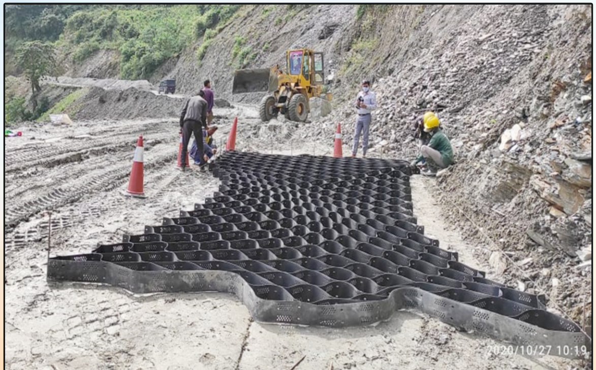
Use of Geocells on Balipara-Charduar-Tawang Road in Arunachal Pradesh
