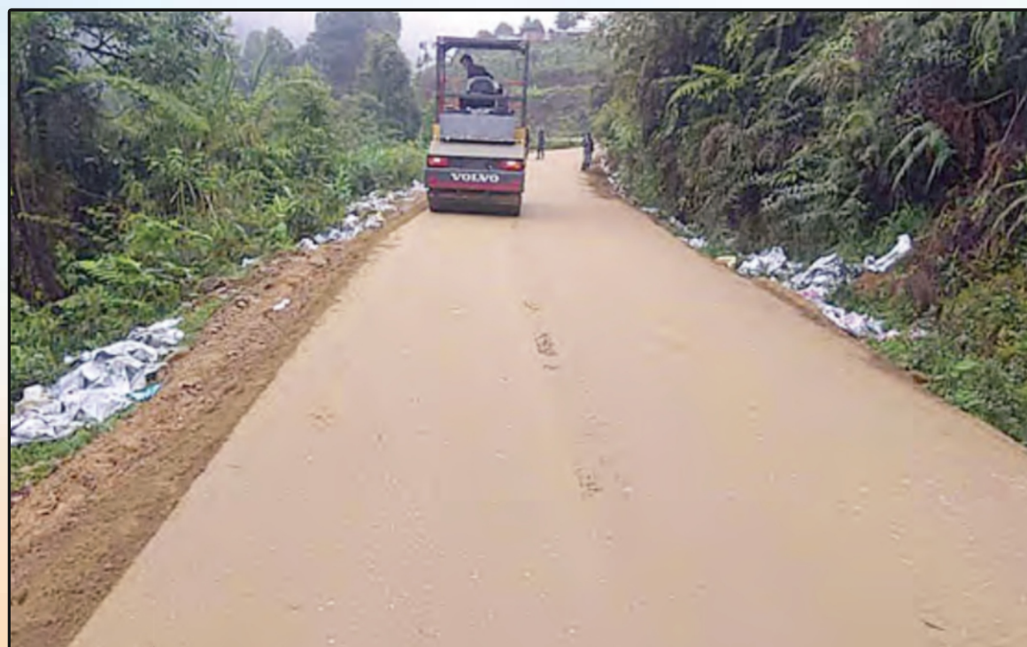
Compacting CTB Layer on Hapoli-Sarli-Huri Road in Arunachal Pradesh
