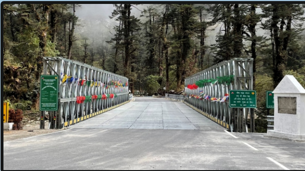
India's First Indigenous CL-70 Double Lane Modular Bridge
