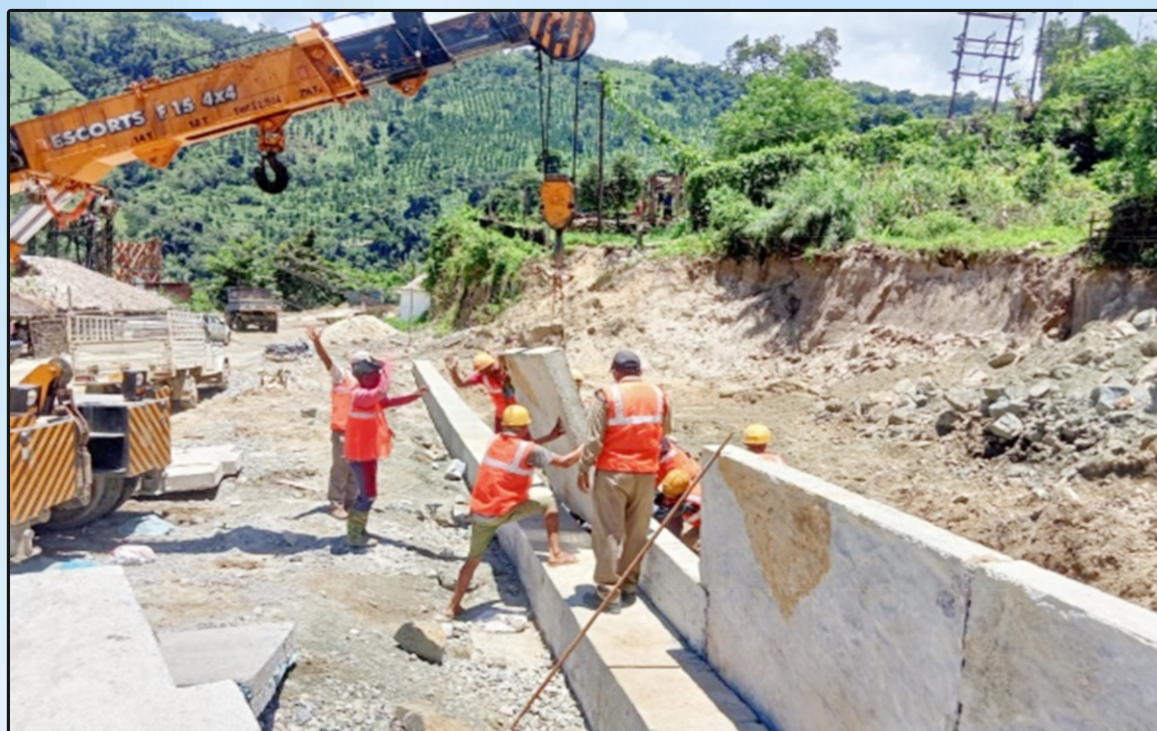
Reinforced Earth Wall Panel Fitting on Along-Yingkiong Road in Arunachal Pradesh
