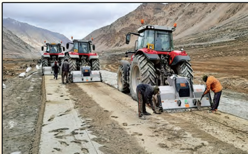
Spreading CT Soil on Mahe-Debring Road in Ladakh
