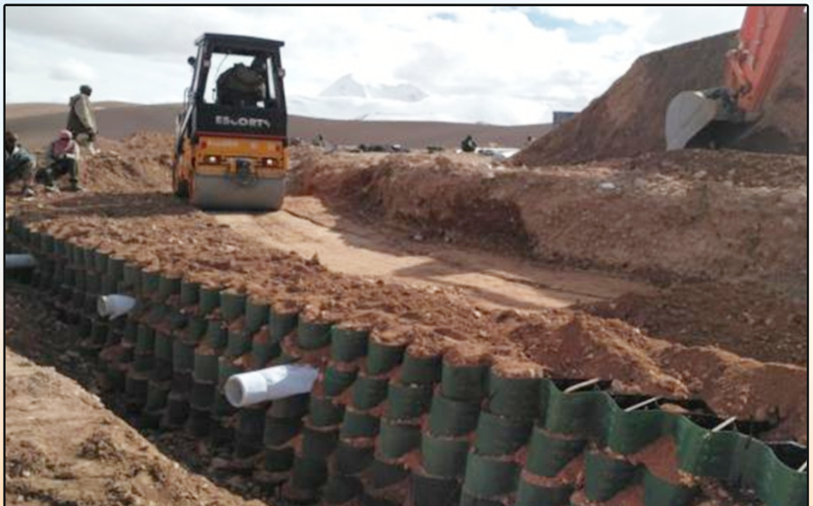
Geocell Works between Km 210- Km 255 on D-S-DBO Road in Ladakh
