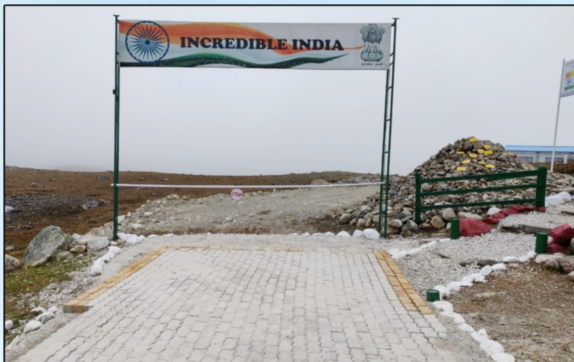
ILCB Pavement on Bumla-Bumla PP Road in Arunachal Pradesh
