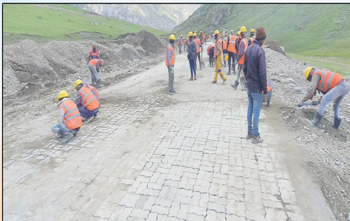
Laying of ILCB Pavement on Srinagar-Sonamarg-Gumri Road in Jammu & Kashmir
