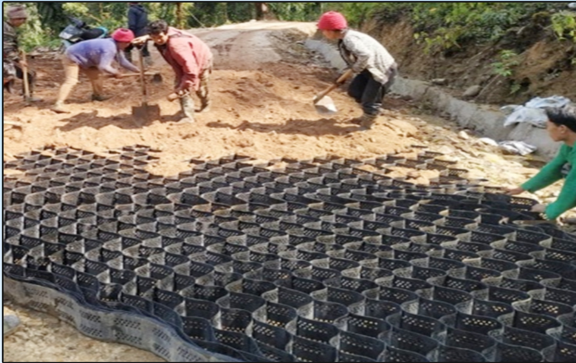
Use of Geocells on Hapoli-Sarli-Huri Road in Arunachal Pradesh
