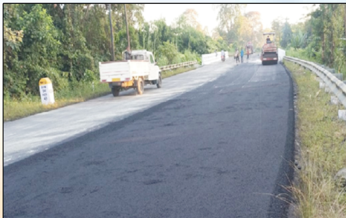
Compaction of Bituminous layer on Roing-Koronu-Paya Road in Arunachal Pradesh
