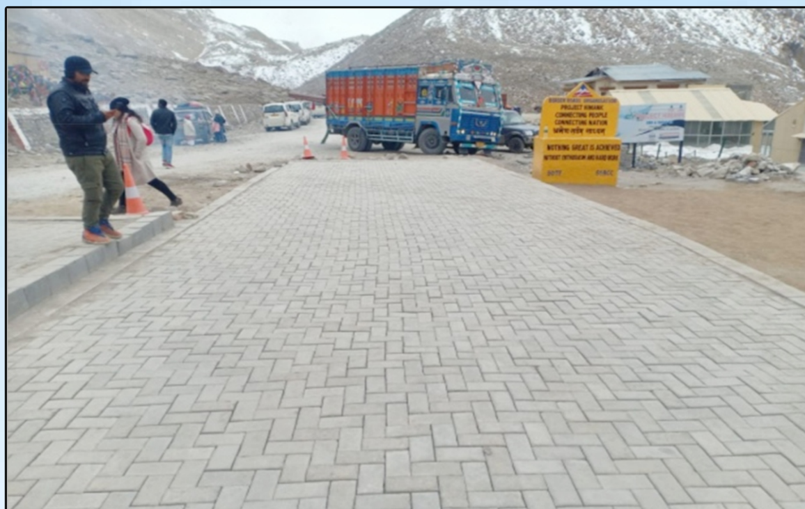
ILCB Pavement at Changla Pass on Karu-Tangtse Road in Ladakh
