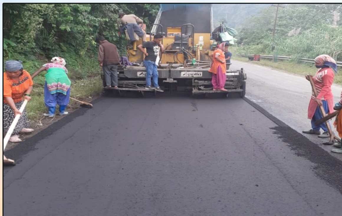
Resurfacing on Balipara-Charduar-Tawang Road in Arunachal Pradesh
