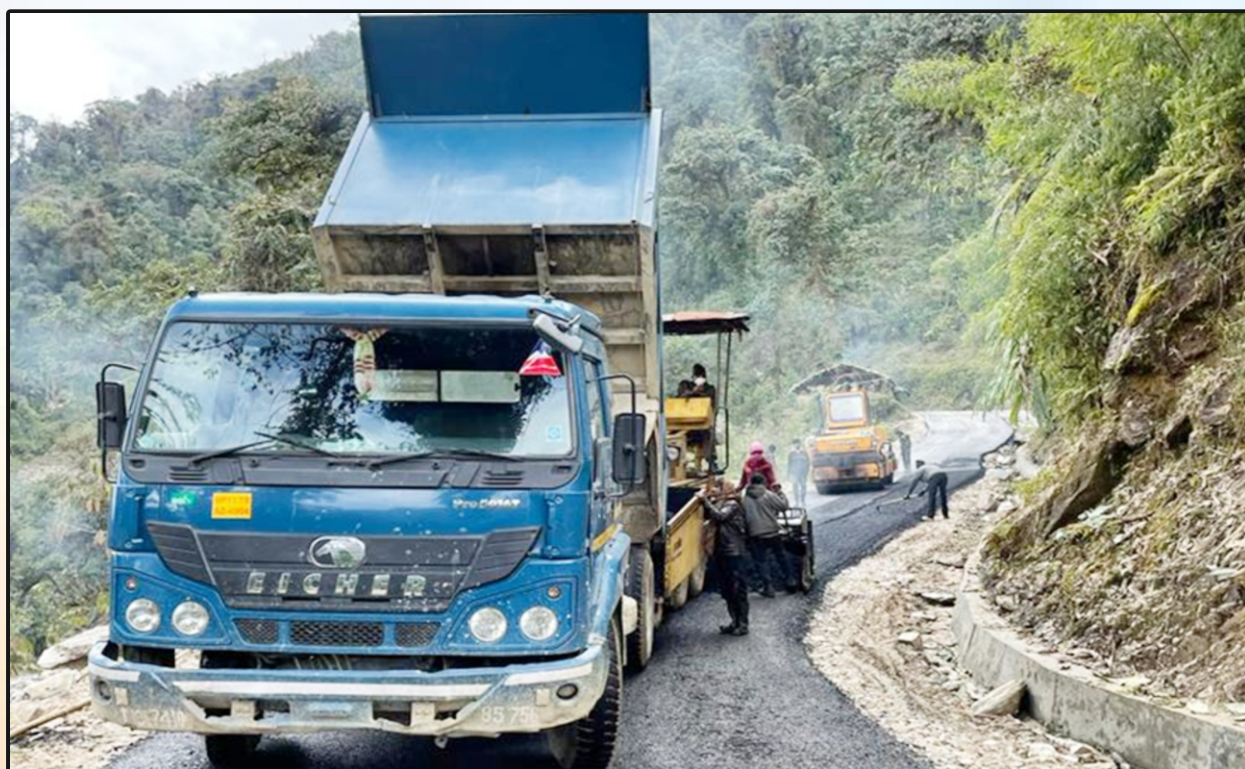
Black Topping Using Plastic Waste on Hapoli-Sarli-Huri Road in Arunachal Pradesh
