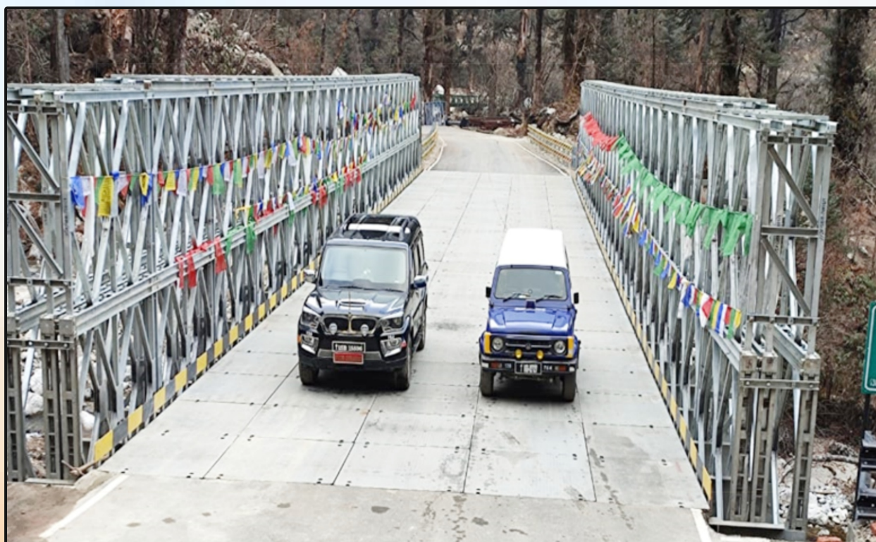
CL-70 Modular Bridge (Double Lane) on Flag Hill-Dokala Road in Sikkim
