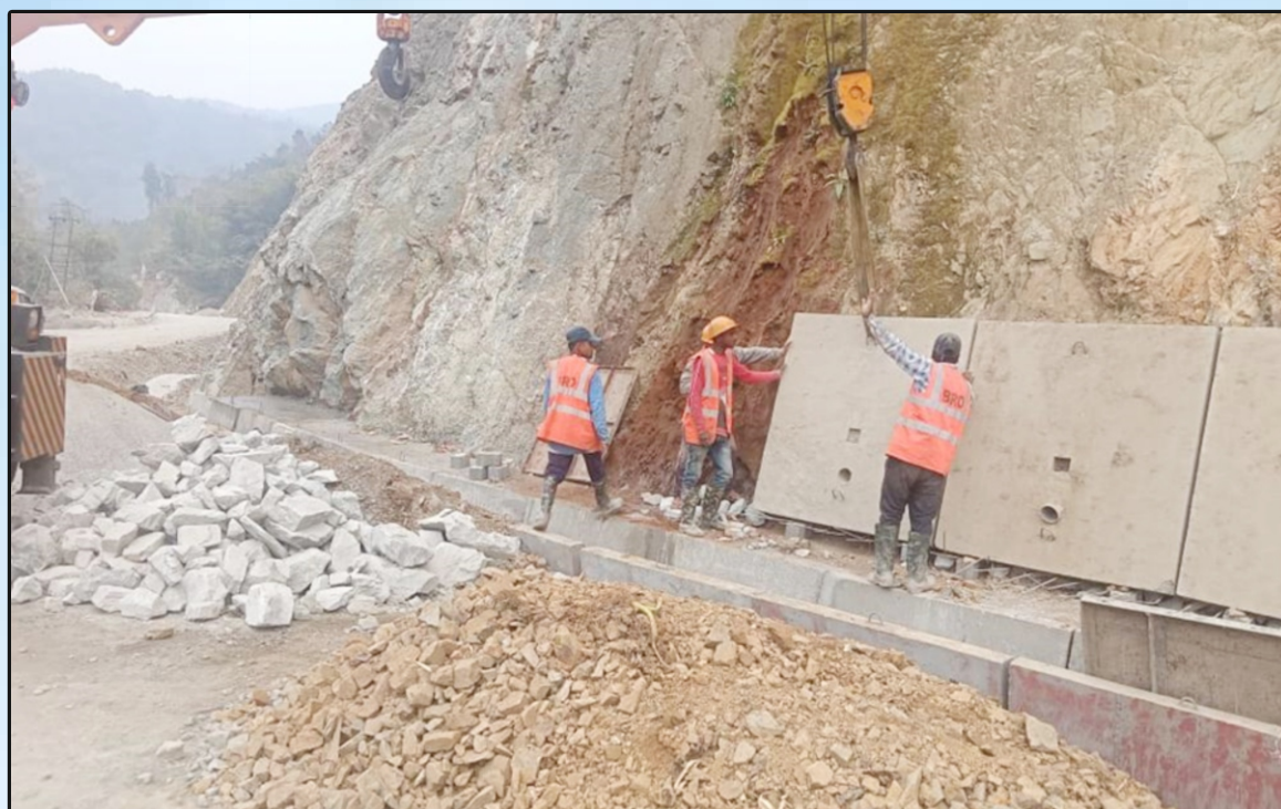
Fixing of Pre-cast Breast Wall on Along-Yingkiong Road in Arunachal Pradesh
