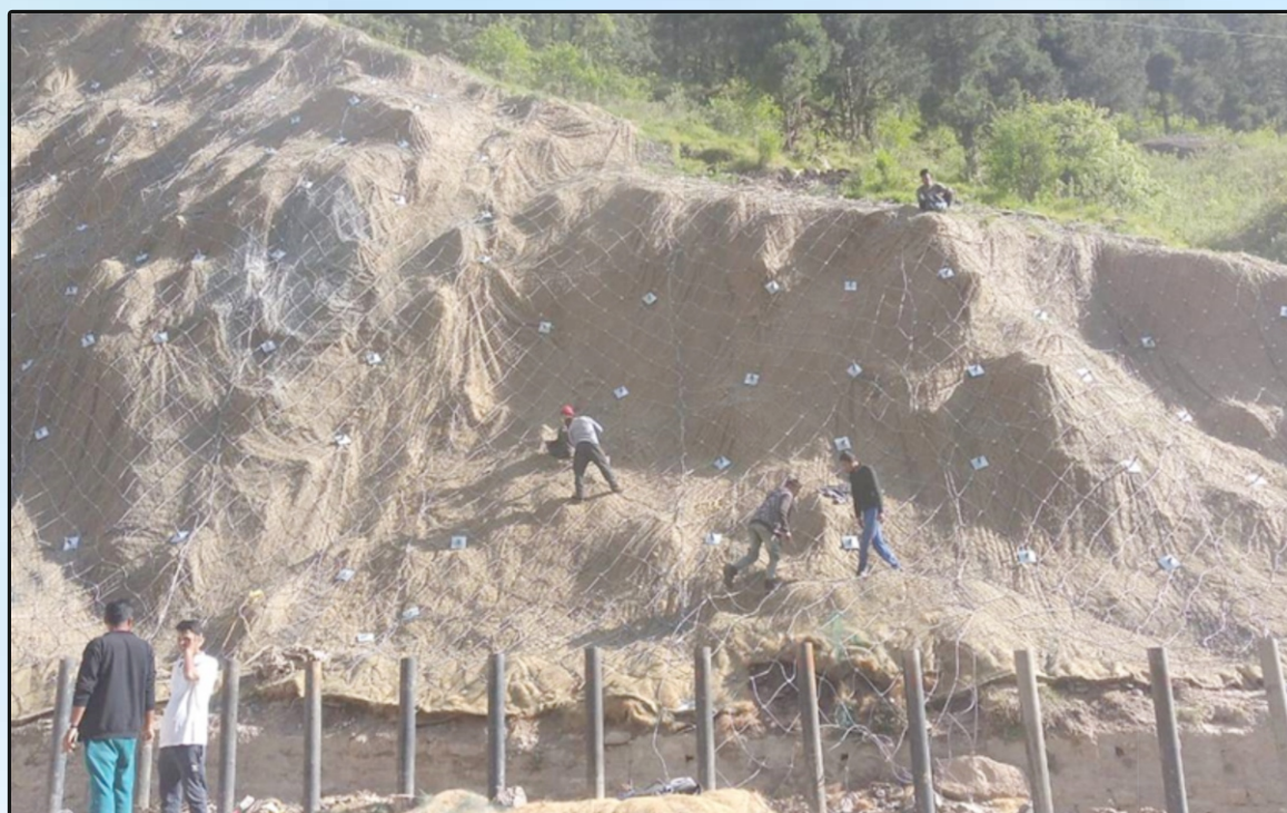
Secured Drapery with Micro Piling Work on Joshimath-Mana Road in Uttarakhand
