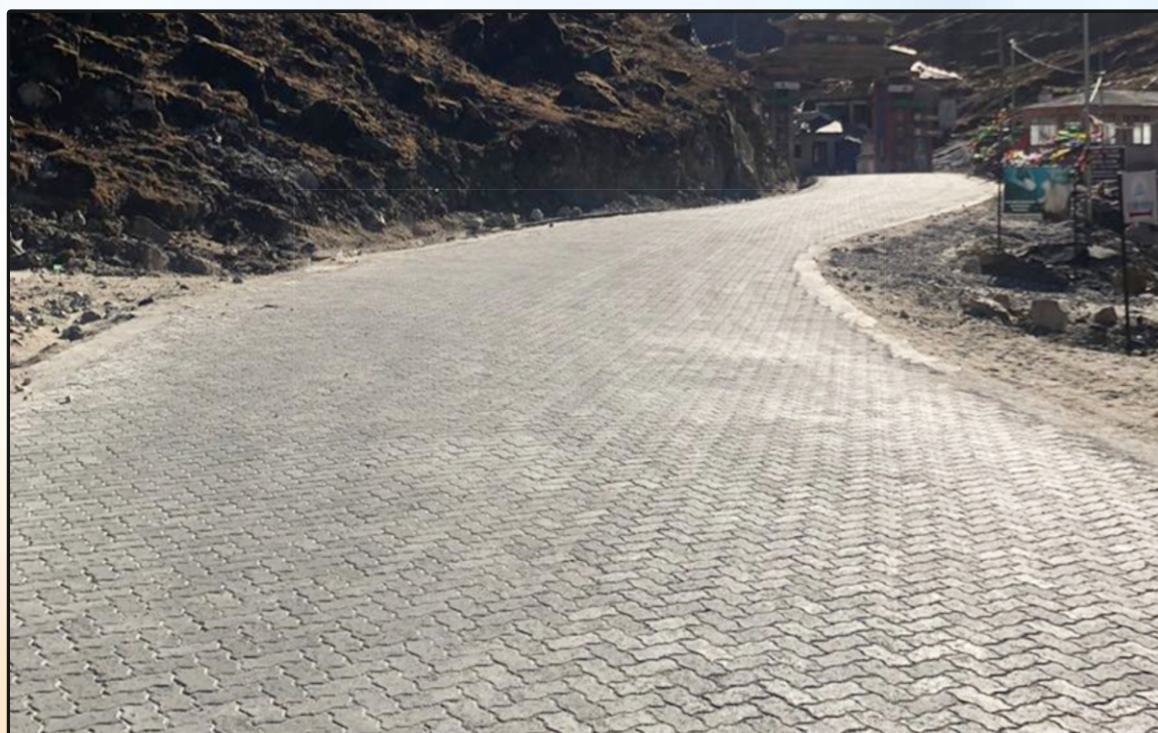
ILCB Pavement on Balipara-Charduar-Tawang Road (Sela Top) in Arunachal Pradesh
