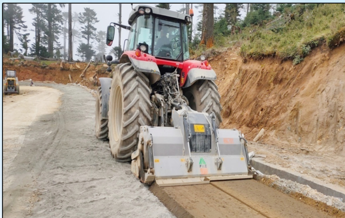
Spreading CT Soil on Mandala-Debrabu-Naga GG Road in Arunachal Pradesh
