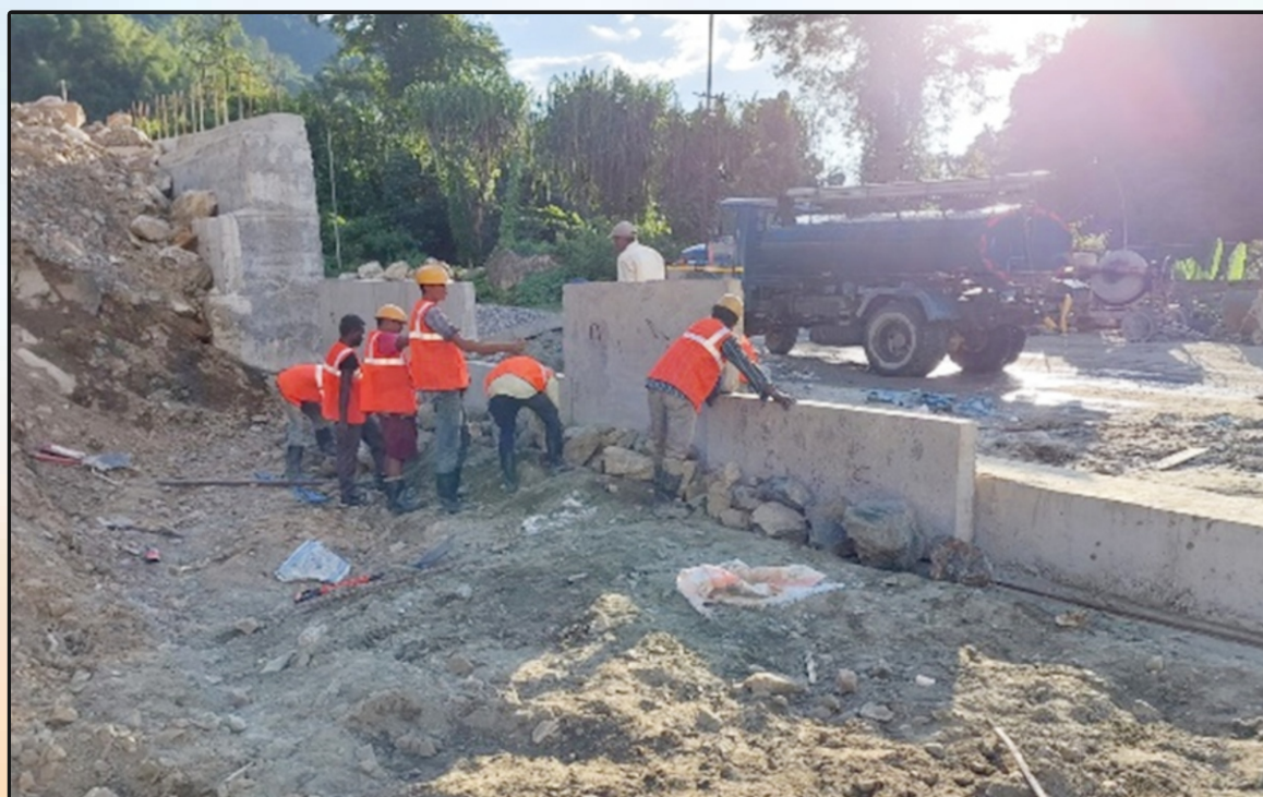
Reinforced Earth Wall under Construction on Along-Yingkiong Road in Arunachal Pradesh
