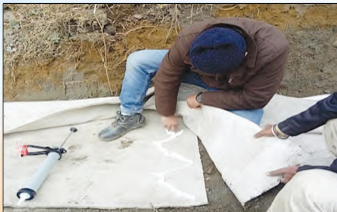
Stage III. Placement & Fixing of Overlap Joints.
