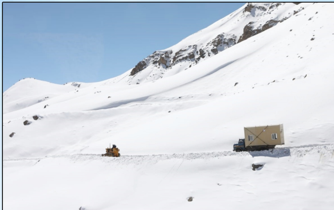
Conveyance of Mobile Containerized Accommodation in Ladakh
