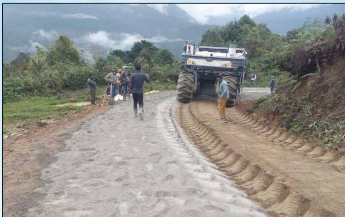
Spreading CT Soil on Hapoli-Sarli-Huri Road in Arunachal Pradesh
