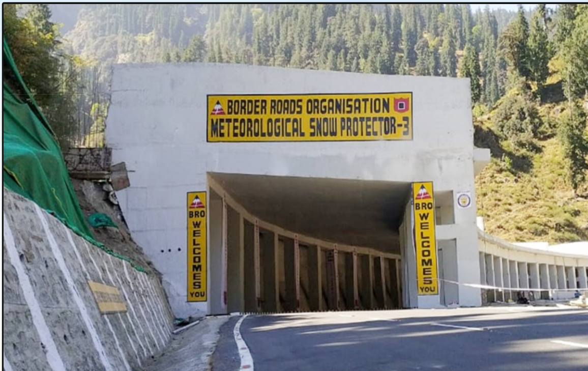
Snow Gallery at Km 4.14 on Approach Road to South Portal of Atal Tunnel in Himachal Pradesh
