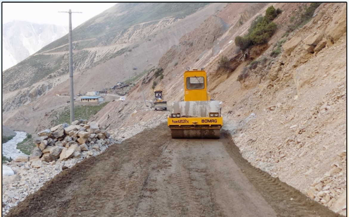
Compacting CTB Layer on Sumna–Rimkhim Road in Uttarakhand
