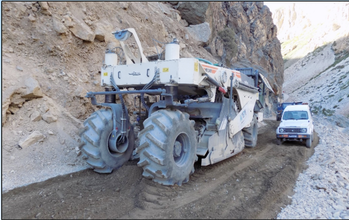
Preparing CTB Layer on Sumna–Rimkhim Road in Uttarakhand
