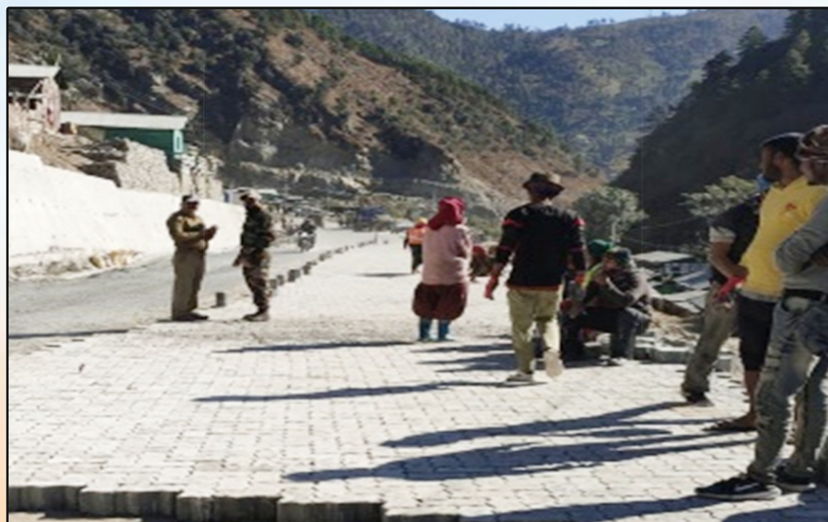
ILCB Pavement on Balipara-Charduar-Tawang Road (Tenga Market) in Arunachal Pradesh
