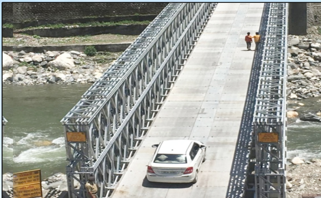
CL-70 Modular Bridge (Single Lane) on Dharasu-Gangotri Road in Uttarakhand
