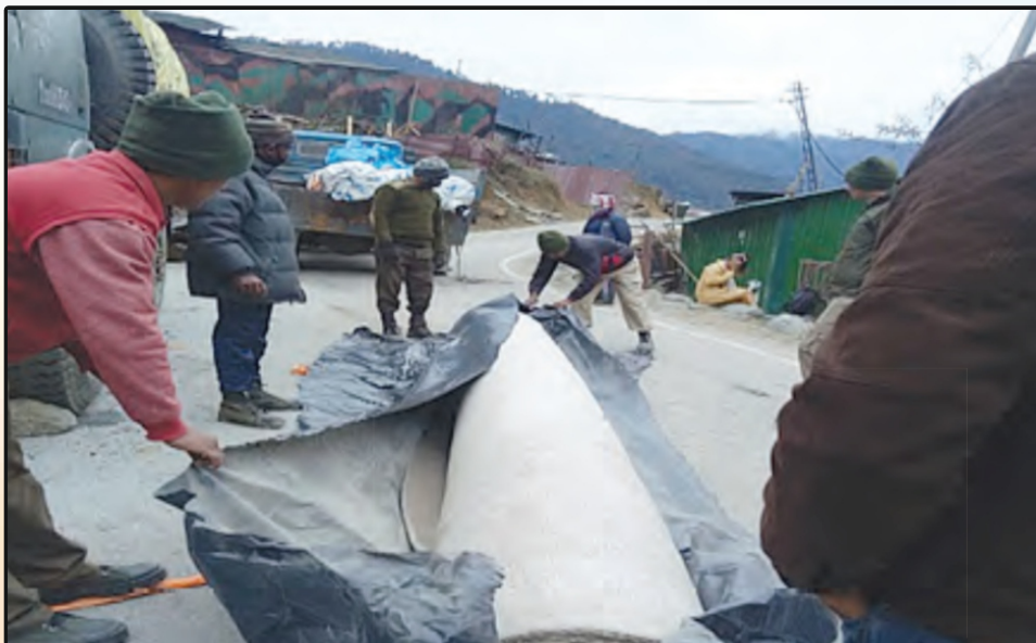
Stage I. Unloading of Sealed Packages.
