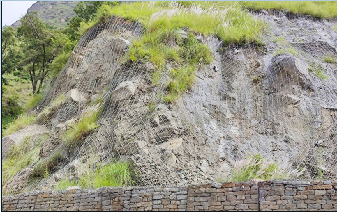
Drapery with Hill Side Gabion Wall on Joshimath-Mana Road in Uttarakhand
