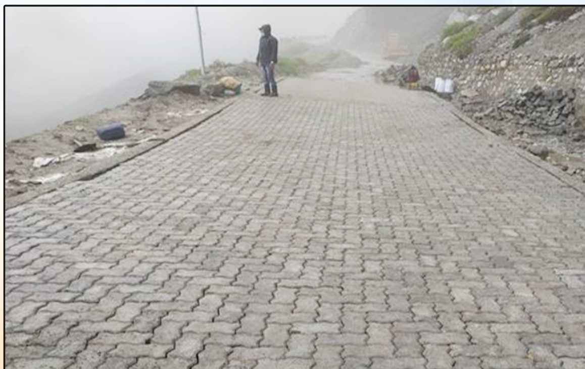
ILCB Pavement on Katao-Bump IV Road in Sikkim
