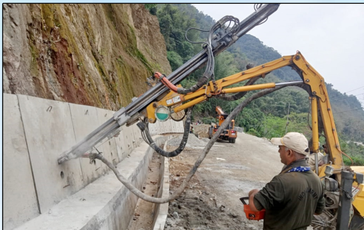
Drilling Pre-cast Breast Wall on Along-Yingkiong Road in Arunachal Pradesh
