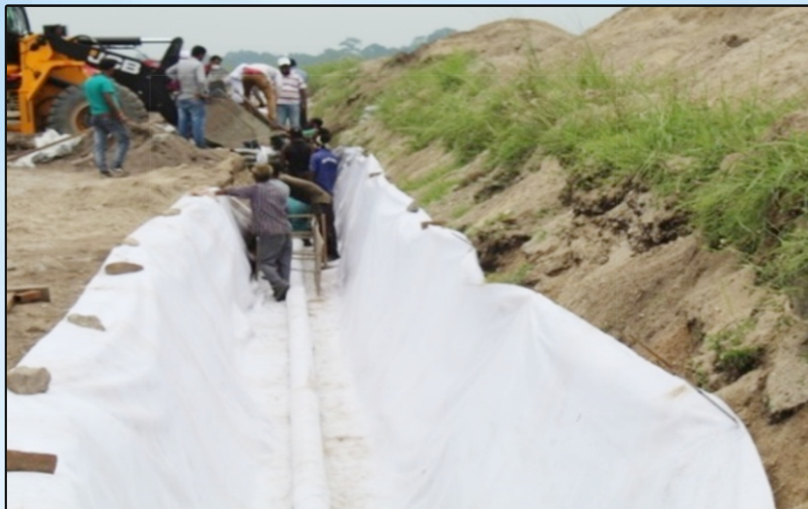
Laying of Sub-Surface Drainage System at Barrackpore Runway in Progress
